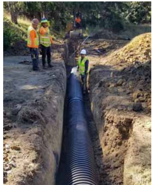
The paving repair at the NFS uncovered some seriously degraded underground culverts! They have been replaced with much-improved versions.
