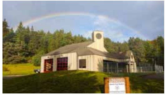
North Fire Station on Highway One.
